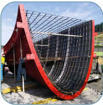
Formwork for trunk-elipsoidal pier. 2014
